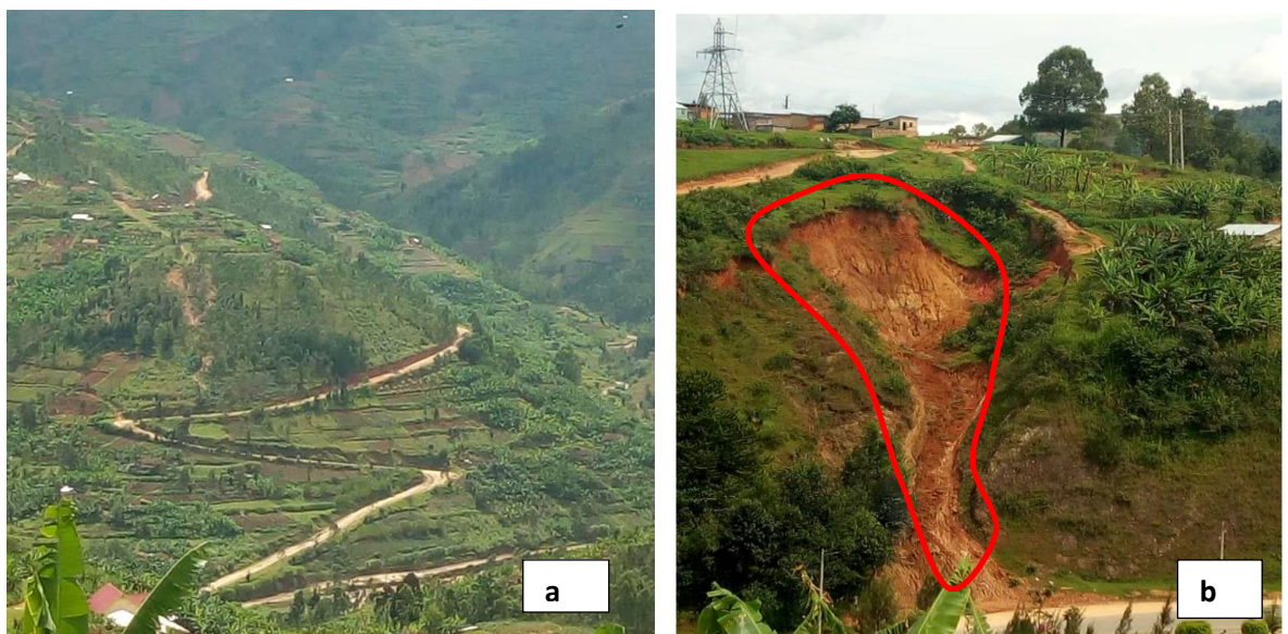
Figure 4 10: Road on steep slope area (a), Landslide on roadside (b)
