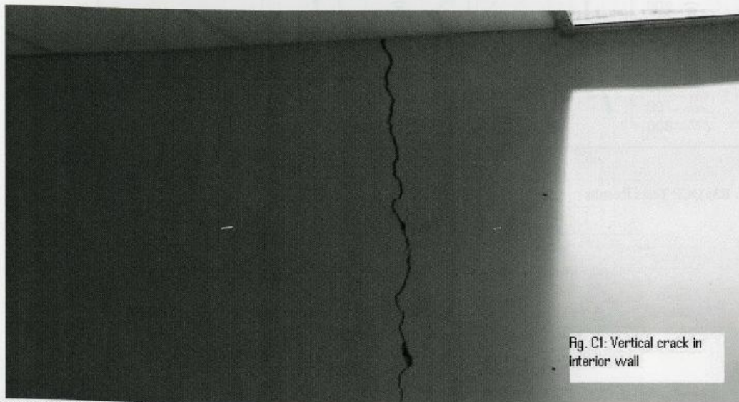
Figure C1: Interior Wall crack
